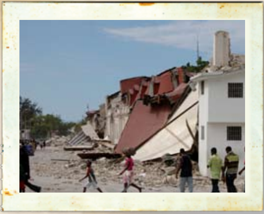
Rescue workers and concerned loved ones continue searching collapsed homes and buildings for more survivors.
